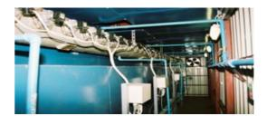
Not only is the pressure low, also the volume is small. But - volume is needed to dislodge the cake from the bag surface. Instead of expensive compressed air we use something which is free: process gas from the clean gas chamber. By right placement of the venturi we get
